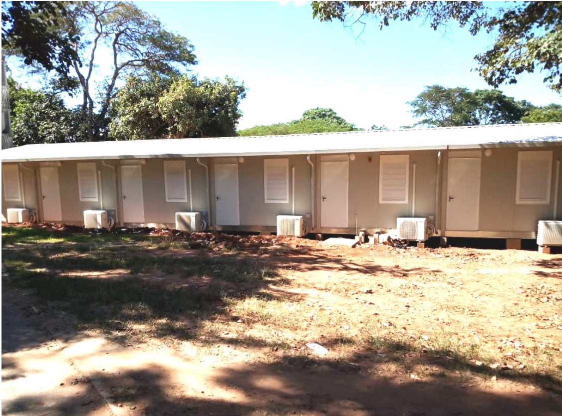
The picture of the Prefabricated Card Production facility in NRB Head Quarter
